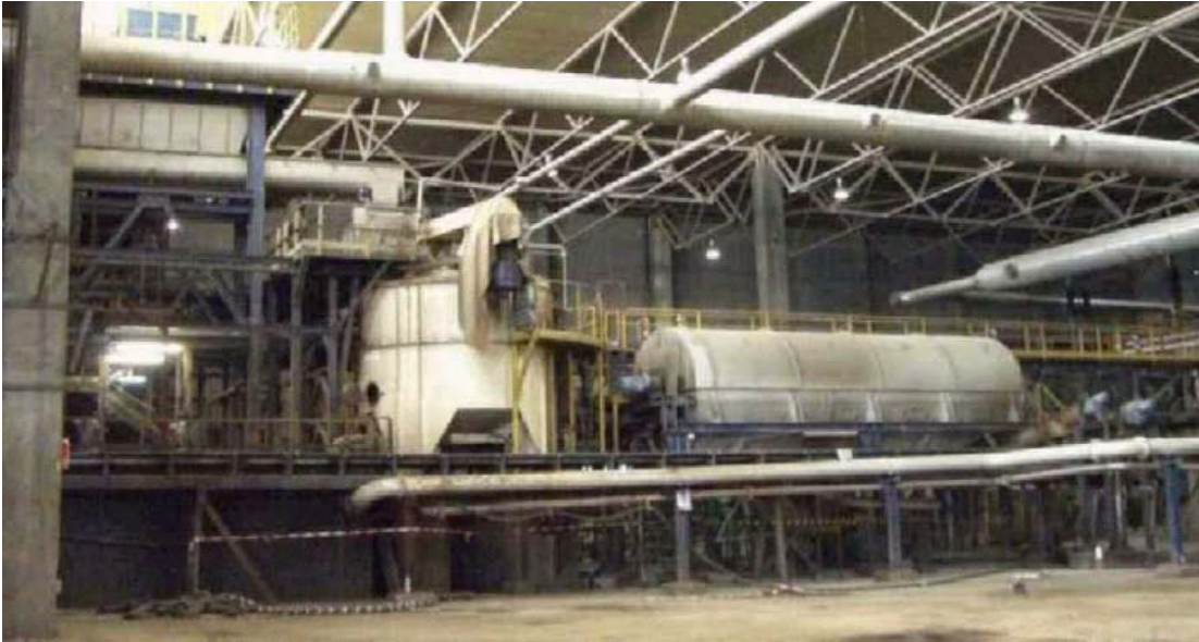
Figure 9 Wet-mechanical processing Ecoparc I (before modification)
