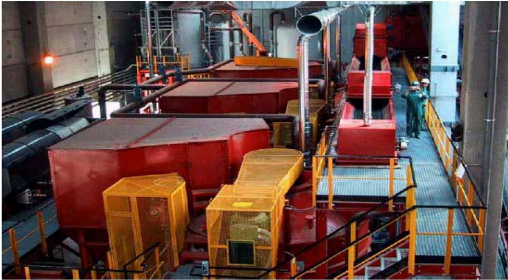
Figure 4 Wet-mechanical BTA processing in Ca' del Bue, Verona – left edge: thickening, in the background: BTA grit removal system
